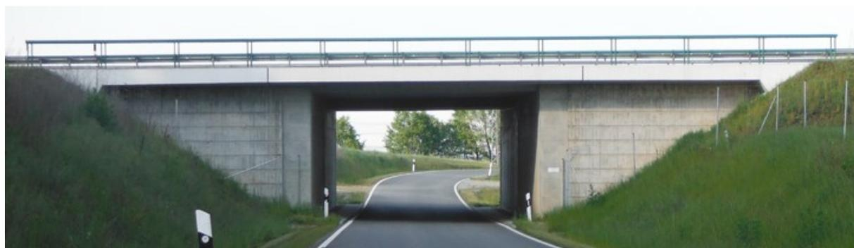
Figure 6. Single-span concrete slab bridge
